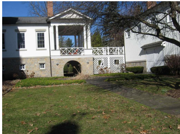
Walkway/porch to Garage
