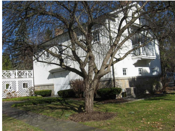
Rear of Garage facing house
