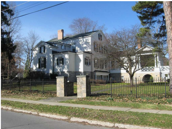
Rear and Right Side (from front) and part of fencing
